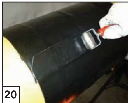
20 Roller the closure patch in the overlapping area. Let the installed closure patch cool down before continuing with application.
