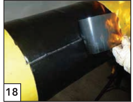
18 Progressively warm along the length of the closure patch and press it on until butyl adhesive is visible out of the side.
