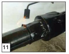
Press the sleeve while warm to ensure full contact with the pipe. The shrinking procedure is finished when the sleeve fits tighly and the thermo-indicator is no longer tangible.
