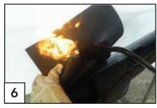
Remove protective film completely, wrap the sleeve around the pipe, heat the inside of the end of the sleeve and close it with overlap..
