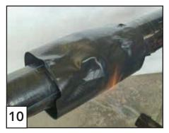
Beginning below, warm the shrinkable sleeve in the middle, moving the torch in a circumferential direction with blue-yellow flame. Next, shrink the spigot side using the same motions. Finally, shrink the socket side. Ensure even shrinkage.
