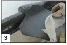
Remove approx 300 mm of the release film from the whole width of the mitred end of the sleeve.
