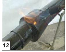
Beginning from the center again, lead the flame to the closing strip in circumferential direction, while shrinking the spigot end.
