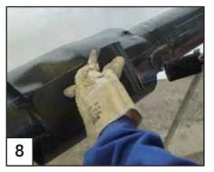
Position the closing patch over the exposed edge of the sleeve. Warm up first one side and press it on.
