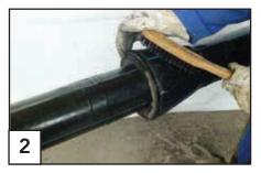
Clean the pipe surface thouroughly to very thouroughly (St 2 - St 3) with a hand wire brush. Remove rust, dirt and other residues.
