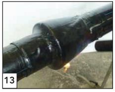
When sufficient temperature is reached, the texture on the sleeve will become smooth. The shinking procedure is finished when the sleeve is tightly fitting everywhere and appears smooth.
