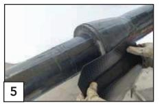
Press the sleeve into place at the 10-or 2-o'clock position in axial direction, overlapping the socket joining evenly on both sides.
